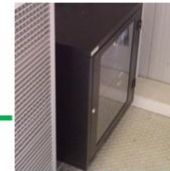
Energy Management System
