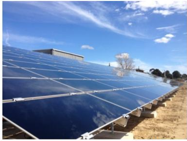
PV : Toucan 5MWc / Test zone 57 kWc
