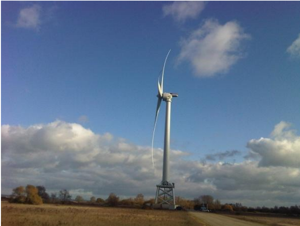
Test of Halliade 6 MW turbine onshore
